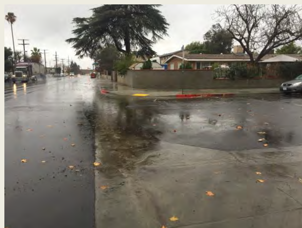
Intersection After Construction
