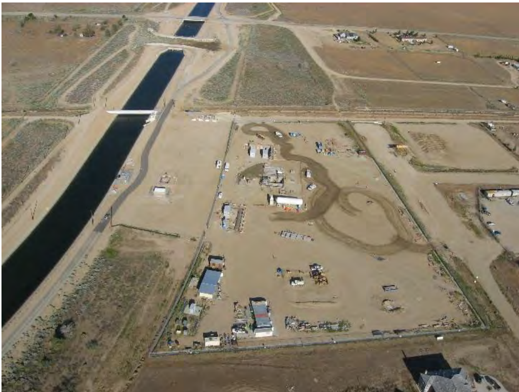
Neenach Temporary Pumping Station, construction site, looking northerly, taken May 4, 2015, by Aqueduct Aerial Patrol.
