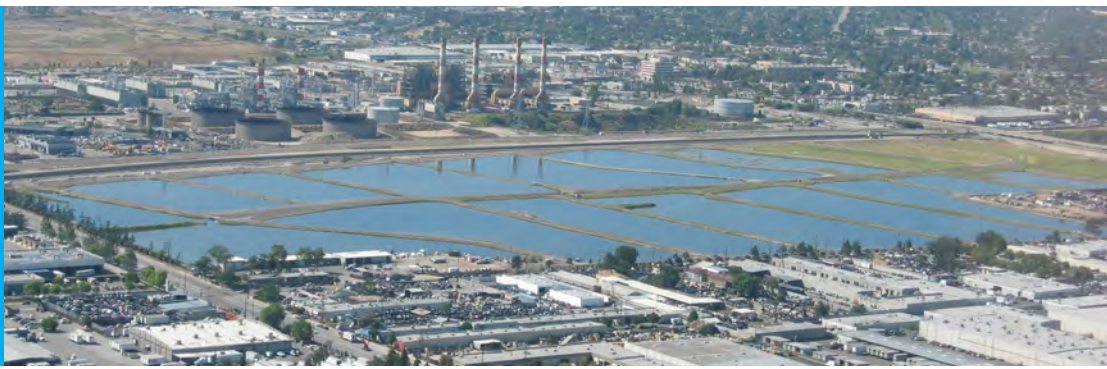
Hansen Spreading Grounds
