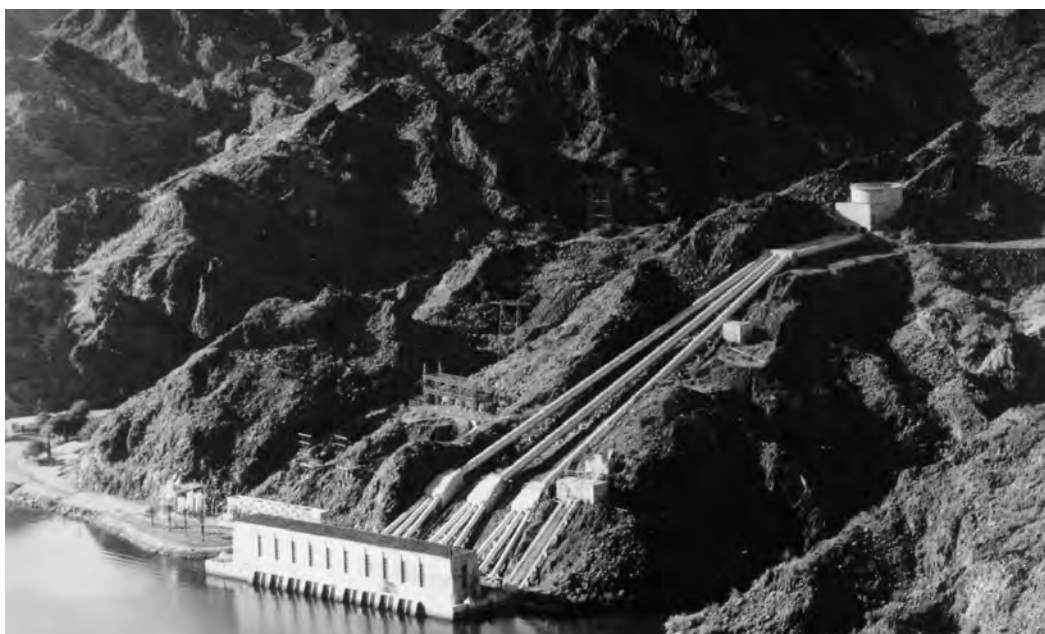
Colorado River Aqueduct Intake - Whitsett Pumping Plant at Lake Havasu, courtesy of Metropolitan Water District
