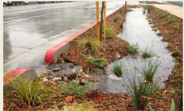
Bioswale along Woodman Avenue Median
